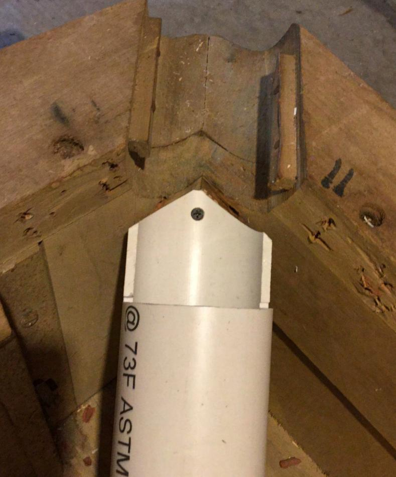
For future dissassembly/ reassembly, uniquely ID mark all the joints. Again, I used no cement. Tap-in snug PVC joint seating provided plenty of structural stability. 4
